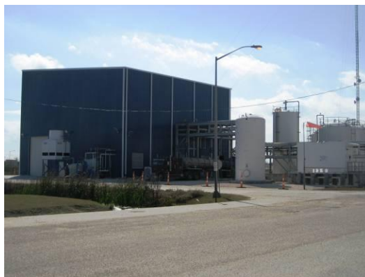
New Deer Park, TX PAC Plant
